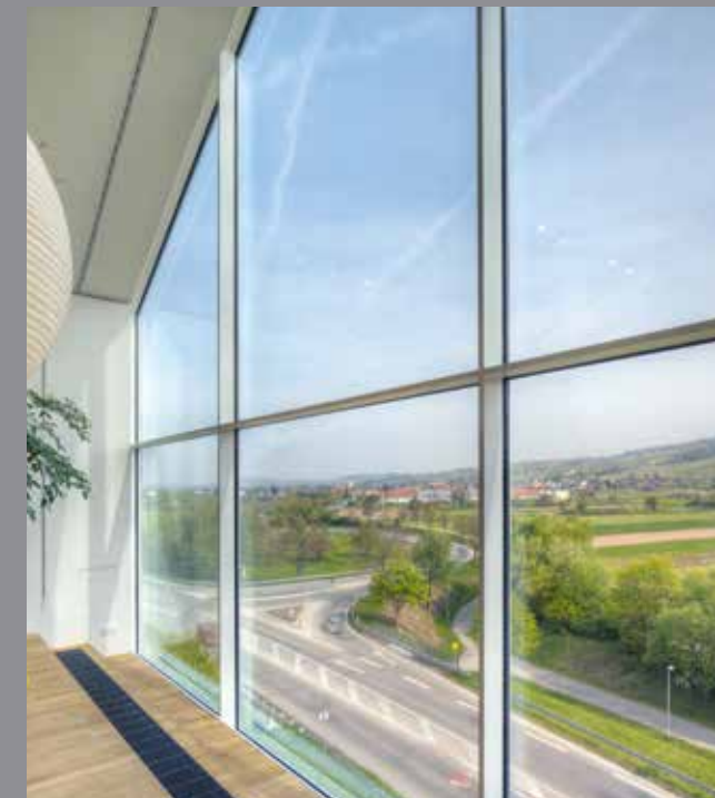
VITRAHAUS, Showroom Interior facades executed using 30 mm / 1.18 in wide steel mullions.
