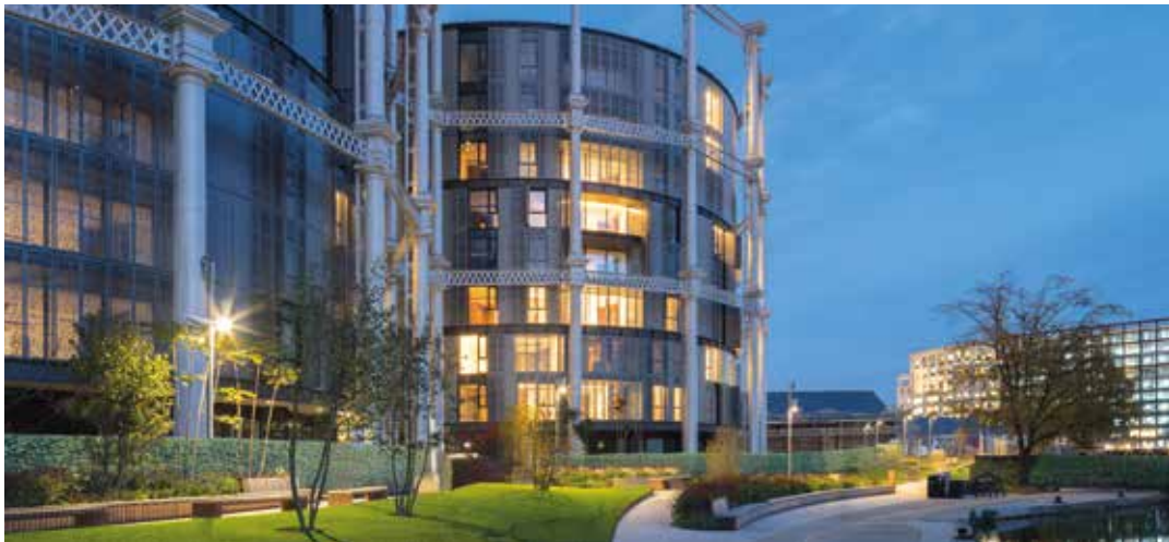
GASHOLDERS LONDON | London, UK WILKINSONEYRE Unitised facade with metal curtain wall featuring integrated motorised concertina blind systems. Sliding doors to steel balconies with glass parapets. Glazed internal courtyards, motorised sliding roofs.
