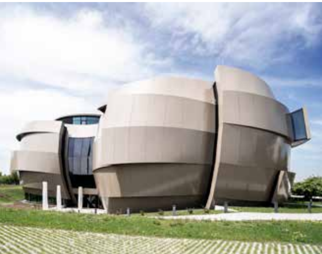
ESO SUPERNOVA | Garching, Germany BERNHARDT + PARTNER 3,200 m 2 / 34,444+ ft 2 of rear-ventilated system facades using 4 mm / 0.157 in aluminium sheet metal panels. 550 m 2 / 5290 ft 2 steel stick system facades with a cupola roof (star roof), diameter 17 m / 55+ ft.
