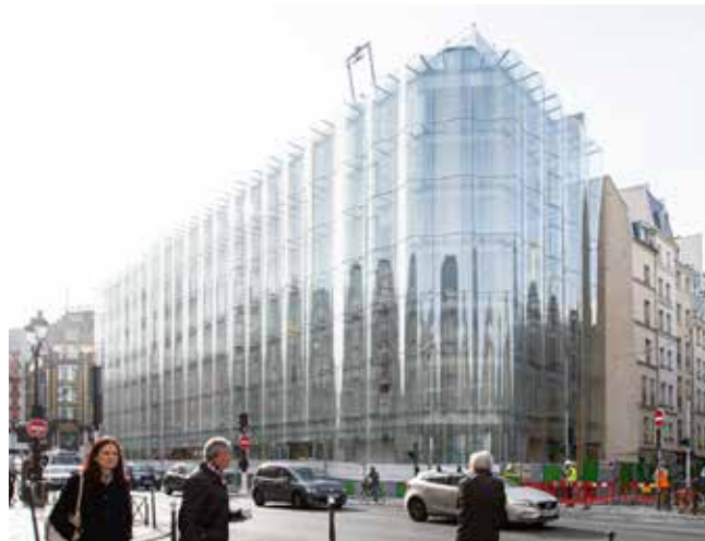
LA SAMARITAINE | Paris, France SANAA Undulating glass facade with graduated mirror print. Facade in white, with white graduated screen print, thermal facade using triple-layer glazing. Patio facade, roof terrace facade, various glass roofs and a pedestrian bridge.
