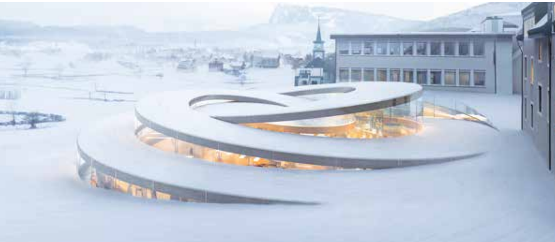
MAISON DES FONDATEURS AUDEMARS PIGUET | Le Brassus, Switzerland BIG, BJARKE INGELS GROUP Load-bearing glass facade comprising over 100 curved, trapezoid glass panels in various formats. Sun protection screen consisting of approx. 15,000 different brass louvres. Steel roof: in the shape of a double helix, using approx. 50 different elements all of which are solely supported by the glass panels. The glazing also makes the building self-reinforcing.
