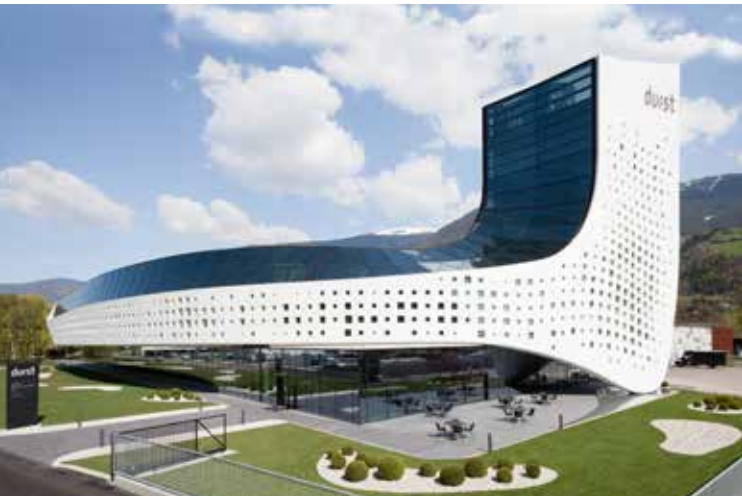
DURST | Bressanone, Italy MONOVOLUME 2,350 m 2 / 25,295 ft 2 freeform metal exterior facade with 850 LED illuminated window elements. 850 m 2 9149 ft 2 triple-layer glazing as skylight strip, comprising approx. 250 panels. 930 m 2 / 10,010 ft 2 stick system facade, 1,200 m 2 / 12,917 ft 2 faceted stick system facade.
