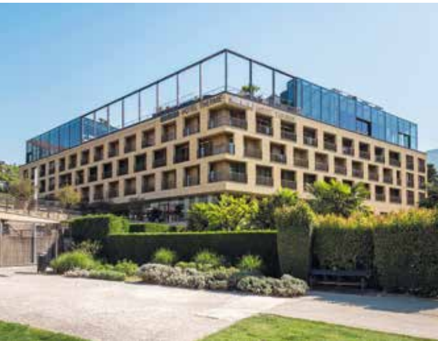
HOTEL THERME MERAN | Merano, Italy HUGO DEMETZ 1,900 m 2 / 20,451 ft 2 wraparound aluminium stick system exterior facade with triple-layer glazing. 1 m / 3+ ft deep and 2 m / 6+ ft wide skylights. All-glass connecting corridor 4 m / 13+ ft high x 3.2 m / 11+ ft wide).
