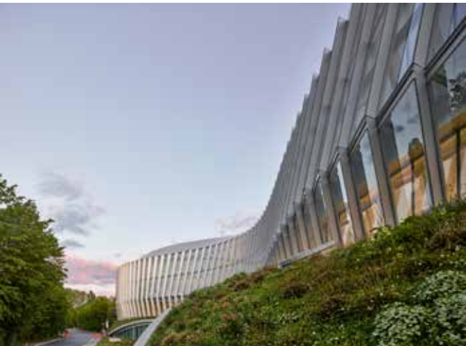
IOC HEADQUARTERS | Lausanne, Switzerland 3XN ARCHITEKTEN Exterior facade: customised 3,100 m 2 / 33,368 ft 2 inclined glass curtain wall, rotated in plan view and consisting of approx. 582 structurally bonded glass panels. Interior facade: 2,300 m 2 / 24,757 ft 2 all-glass facade with silicone joints.
