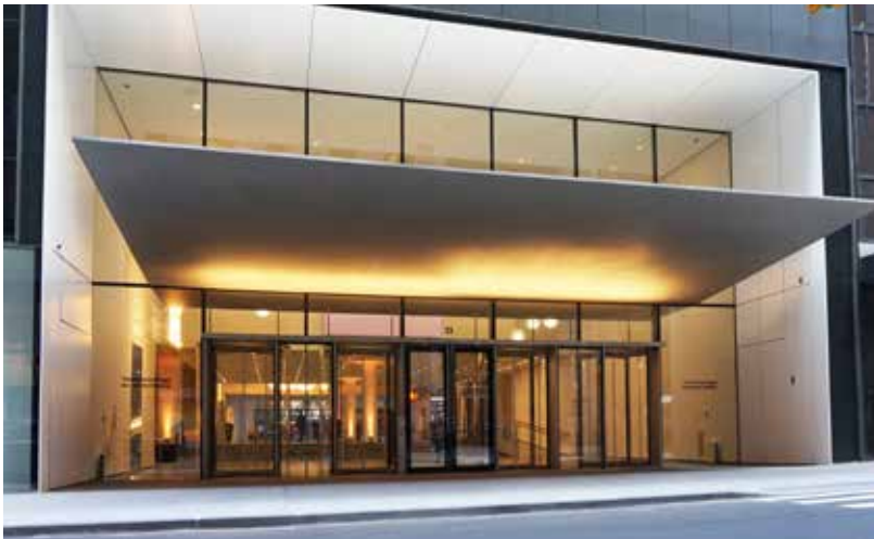
MOMA | New York (NY), USA DILLER SCOFIDIO + RENFRO 360 m 2 / 3875 ft 2 entrance facade with metal cover panels, cantilevered entrance canopy 20 x 7 m / 65+ x 23 ft with glass bead blasted surface, delivered to site in 3 parts. 215 m 2 / 2314 ft 2 of ground floor shop facades and 350 m 2 / 3767 ft 2 tension rod facade, 590 m 2 / 6350 ft 2 panel facade.
